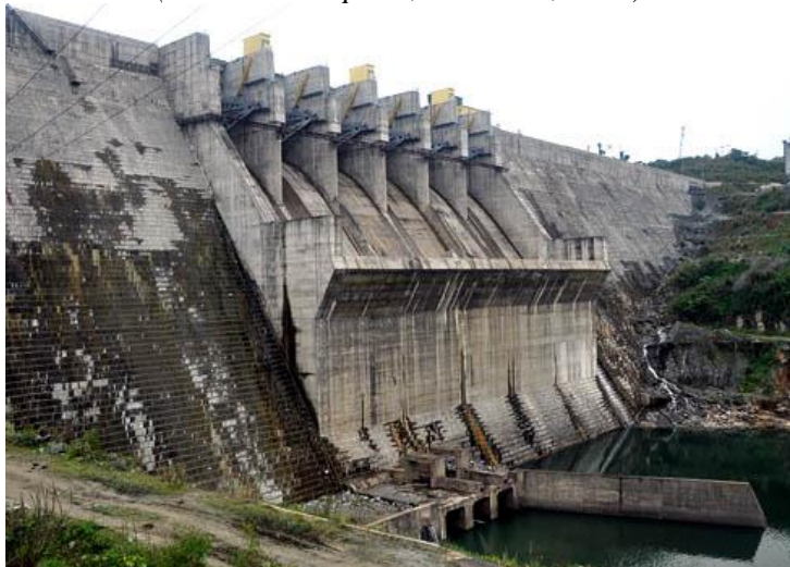
Figure 9 - Water leaks through Song Tranh 2 dam in March 2012 (Source: VnExpress, March 28, 2012)
